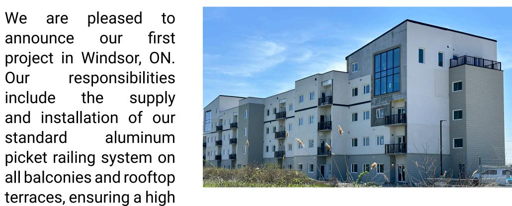
We installed approximately 800 linear feet of railing on this project, providing both safety and an aesthetically pleasing design to the surrounding area.
