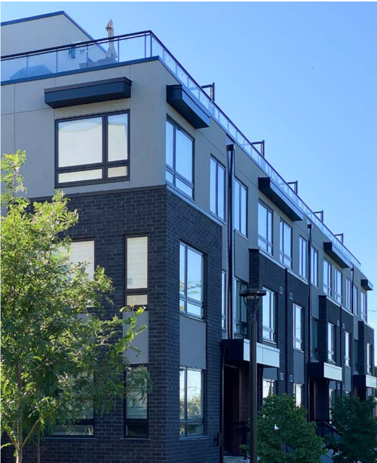
Aluminum frame w/ continuous handrail and tempered clear glass infill. Toronto, ON.
