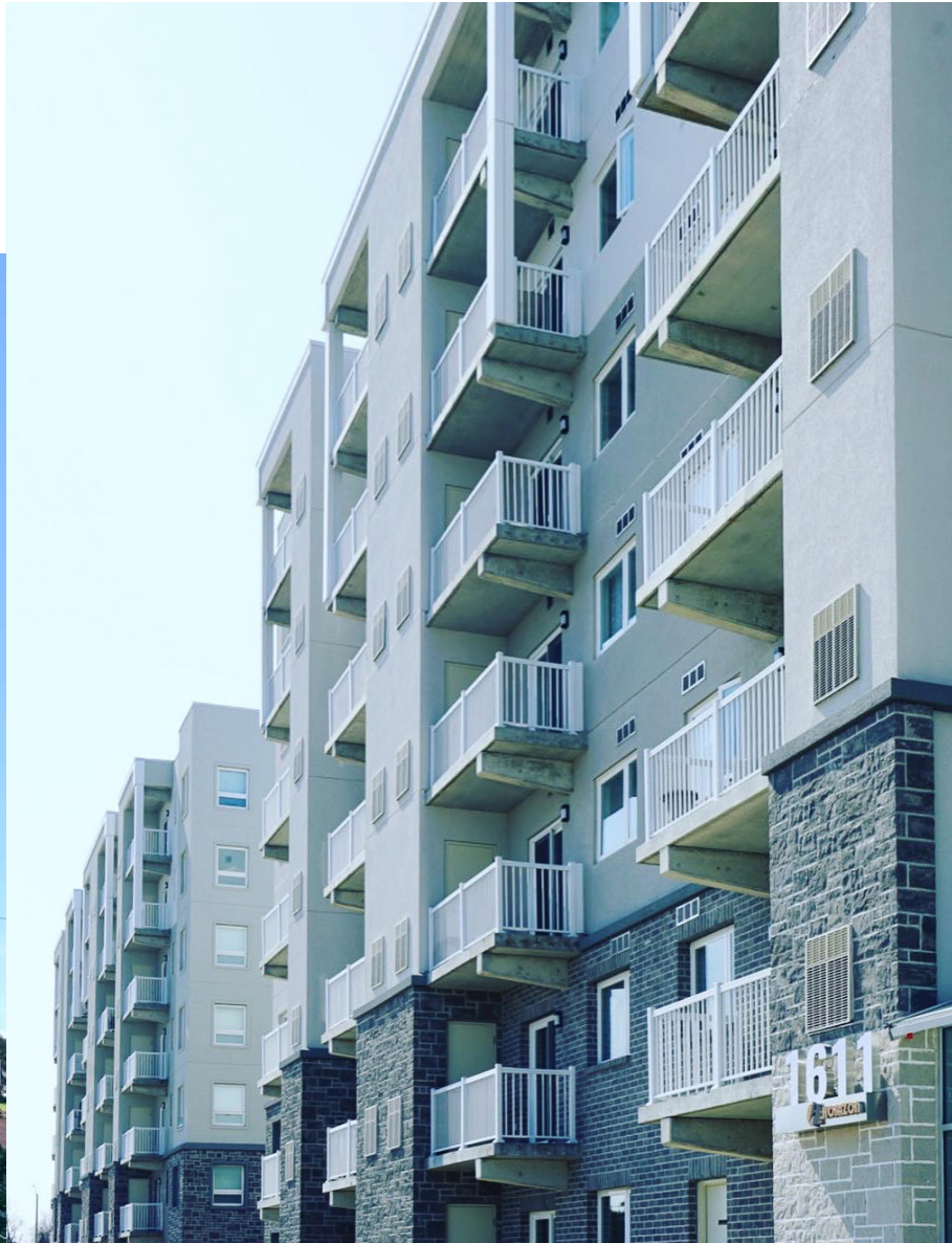
Aluminum picket railing installed on this 7 storey condo building. Windsor, ON.
